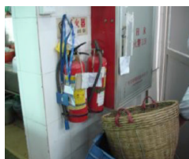
Example of blocking of fire equipment.
